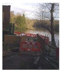
The new footbridge will be installed in the next few weeks. Repair works have been carried to the existing bridge abutments together with some modifications to accommodate the new, narrower footbridge.
