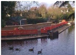
The reinforced concrete floodwall is complete. It has been almost entirely brick clad, the only outstanding section being near the footbridge which will be completed shortly. Following this coping stones will be installed and the floodwall will be complete.
