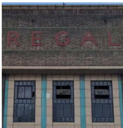
Left: Detail of the original faience 'REGAL' tiles on the frontage, as well as the cream and turquoise window surrounds.
